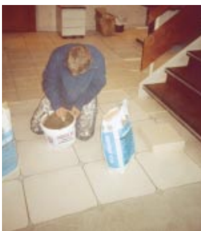
Mixing Ardurit S38 floortile bedding mortar
