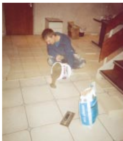
Fluid pourable Ardurit S38 being applied to existing primed floor tiling
